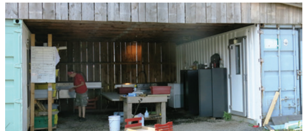
This packhouse is covered to protect produce. All clean produce-contact surfaces are stainless steel or washable hard plastic. A sanitizer is used to clean all surfaces before each wash-pack. Potable well water is used for triple-rinsing produce with a food-safe sanitizer in the first and last washes. Tianna DuPont, Penn State Extension
