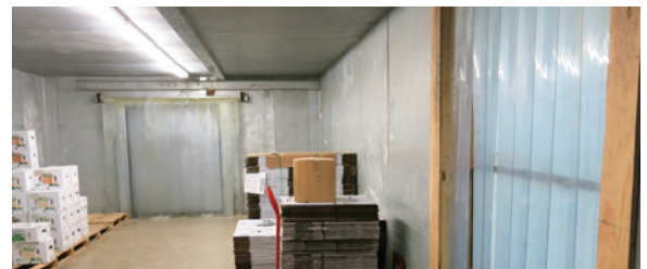
Plastic curtains on doors help retain cold air and save energy. Tuscarora Organic Growers
