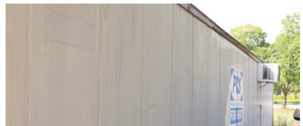
Insulated shipping container retrofitted with a cooling unit to provide produce storage. Roots to River Farm
