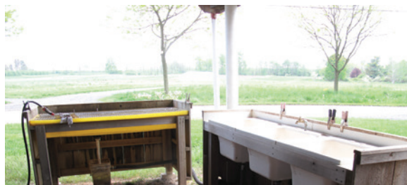
Plastic laundry basins (right) can be plumbed to function as triple-rinse sinks that can be sanitized easily. Penn State Extension
