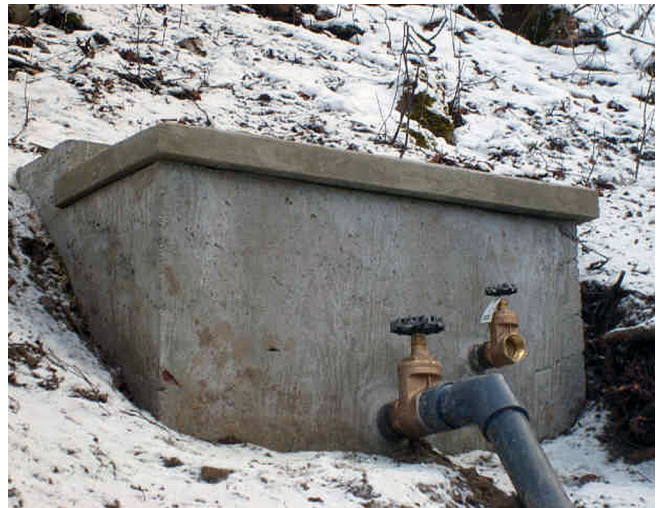
Figure 2. A properly sealed spring box will prevent surface water, insects and small animals from gaining access to the spring. Source: http://aquariusump.com/springbox.aspx .
