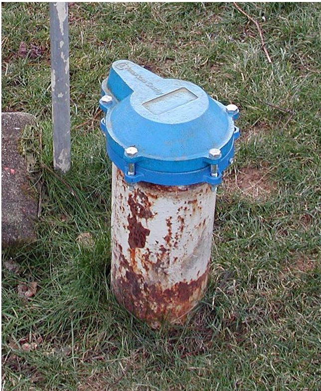
Figure 1a. Properly constructed, drilled well with a sanitary well cap. Source: Bryan Swistock, Penn State University.
