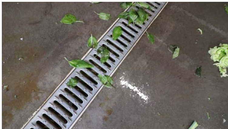
A removable coarse grate on this trench drain helps keep larger debris out while allowing water to pass.
