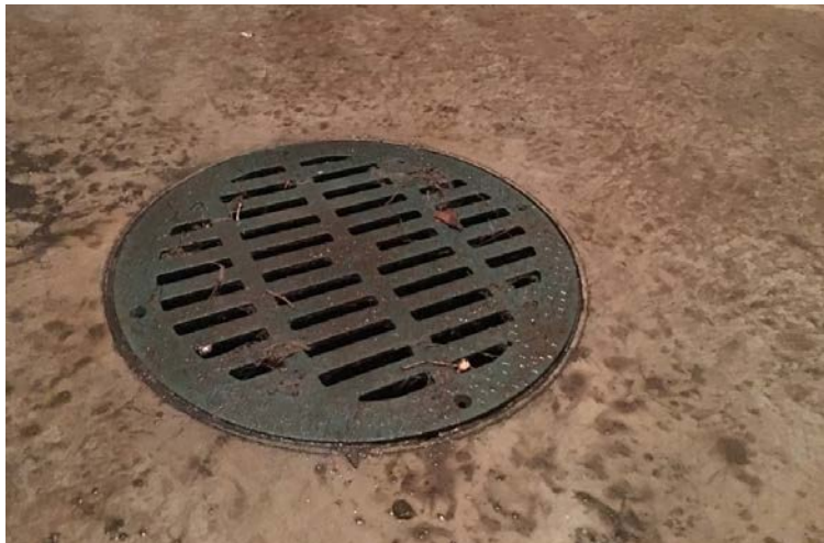
This large floor drain in a cooler is approximately 12" in diameter and serves as a sump or floor sink. It has a larger volume below the grate to serve as catchment for high instantaneous flows of water when the space is hosed down.
